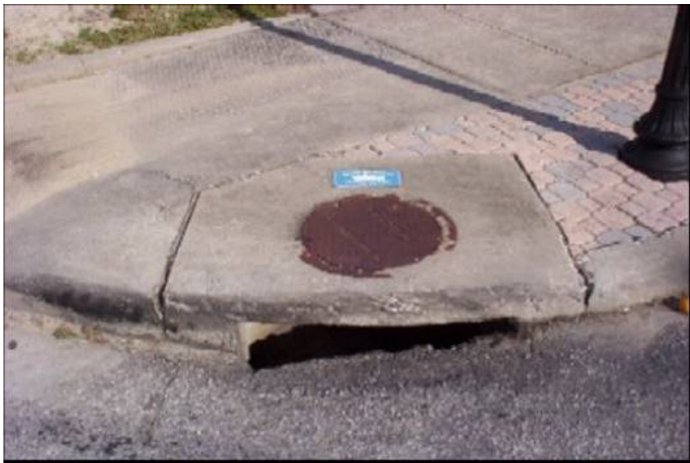
Figure 1. Roadside storm water entrance to a ditch
