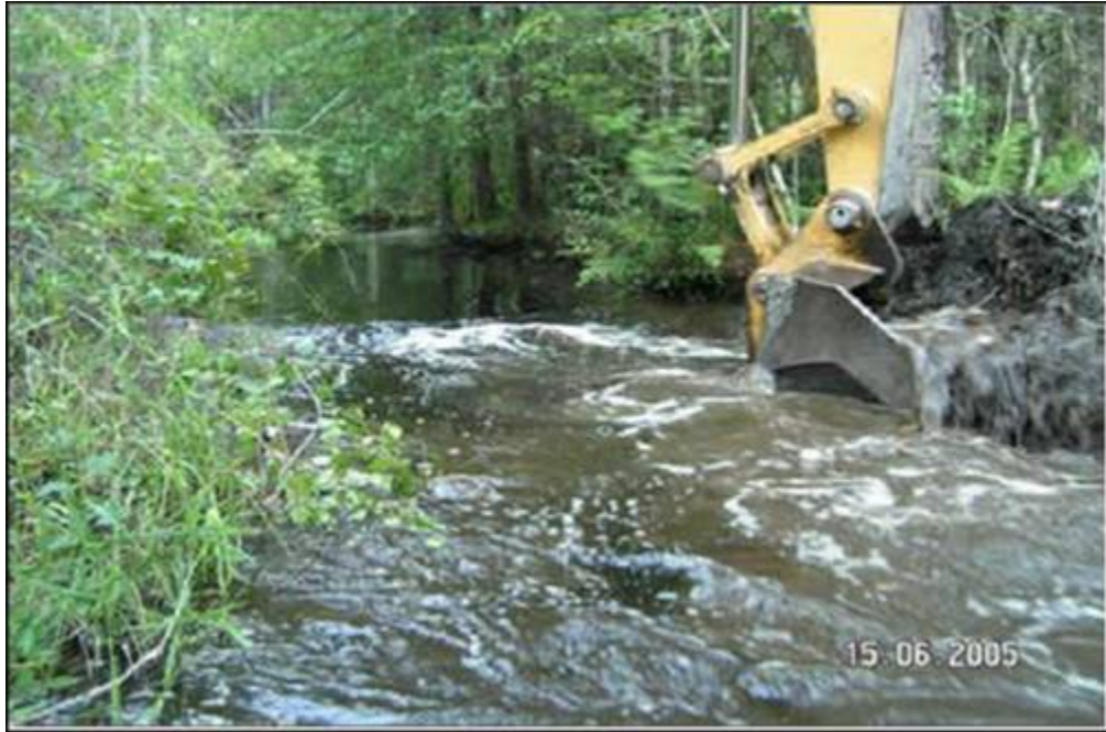
Figure 4. Ditch cleaning operation in by Bradford county public works
